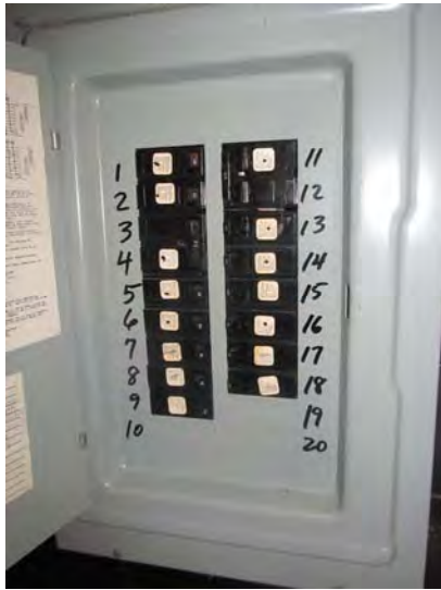
Typical electrical load center with circuit breakers found at each unit – No problems observed or reported
