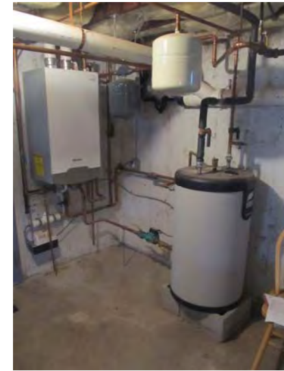
Typical natural gas-fired wall-mounted boiler and indirect-fired domestic hot water tank – All equipment installed as part of recent renovation work
