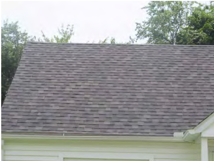
Architectural shingles installed on all roofs as part of recently completed renovation work
