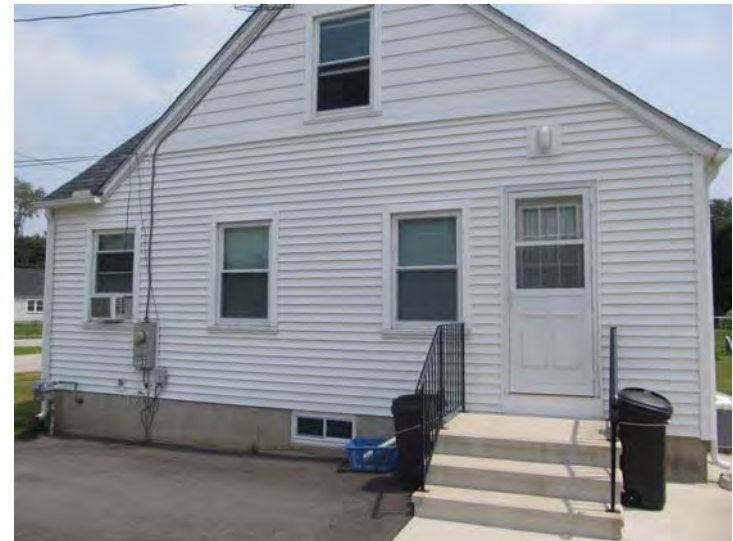
Vinyl, siding, entry doors, storm doors, and windows all replaced as part of recently completed renovation work
